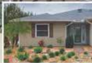
Vinyl Siding Installation
