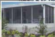
Screen Enclosures & Repair
