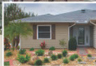
Vinyl Siding Installation
