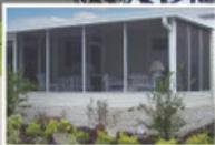
Screen Enclosures & Repair
