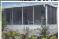
Screen Enclosures & Repair
