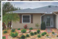
Vinyl Siding Installation
