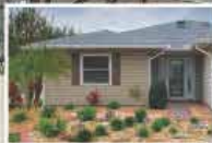
Vinyl Siding Installation
