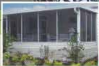
Screen Enclosures & Repair
