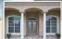
Window & Door Replacement
