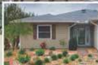
Vinyl Siding Installation
