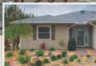
Vinyl Siding Installation
