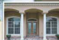
Window & Door Replacement
