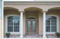
Window & Door Replacement
