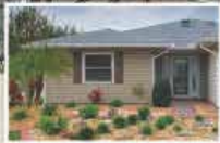
Vinyl Siding Installation
