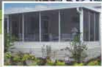
Screen Enclosures & Repair
